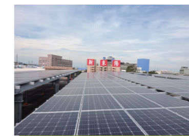
Dayuan Plant solar panels / Dayuan Plant power generation
